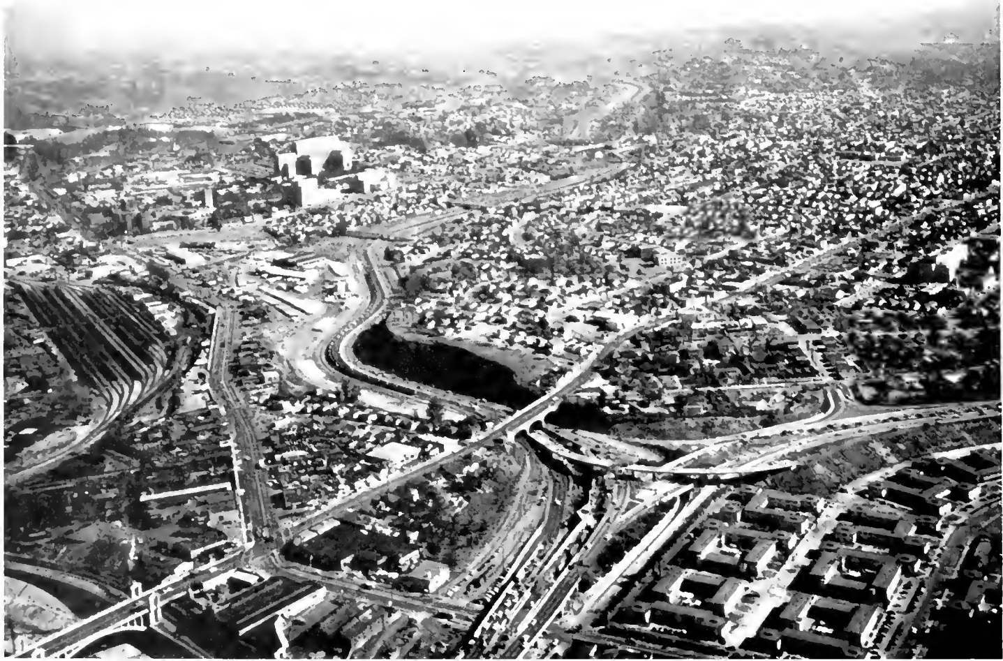
Looking easterly along San Bernardino Freeway from above City of Pomona with Ganesha Park in foreground left and Gorey Ave., State Sign Route 71, in center.
